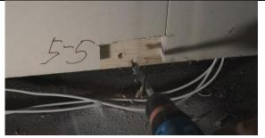
Drilling hole with 10 mm diameter and approx. 20 mm depth.
