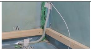
Attach the protector to the wall via tape or plastic hooks. Sensor is at the bottom part. Upper part remains above the floor level in the wall for future possible inspection.
