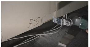
1. Open the wall for sensor installation (use of crown drill bit possible).
