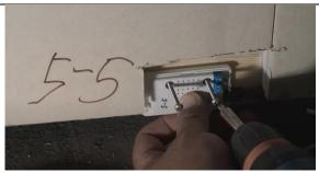
7. Attach the sensor to the wood with bigger screws.
