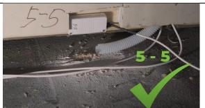
10. Insert protector tube to the wall next to the sensor. This will serve for possible future inspection.
