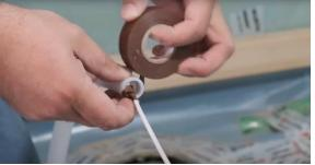
Attach the cable with tape on the other side of protector. Sensor has to be fixed in the protector.
