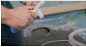
Cut off surface of plastic protector so small ventilation holes appears in the sides.
