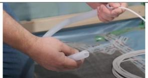
Insert sensor with cable attached to the protector. Sensor has to be in the area of ventilation holes of the protector.
