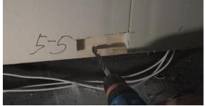
3. Hole for the basket has to be placed such the electrodes of sensor are closer to the middle of timber beam.
