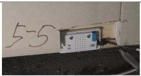
8. The screws has to be driven all the way. Firm attachment of the sensor is crutial.
